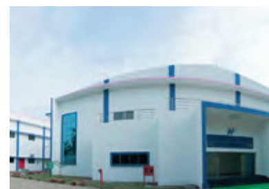
Unipill Block, Kanagala
