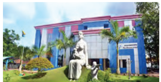
HLL's Corporate headquarters at Thiruvananthapuram, Kerala.
