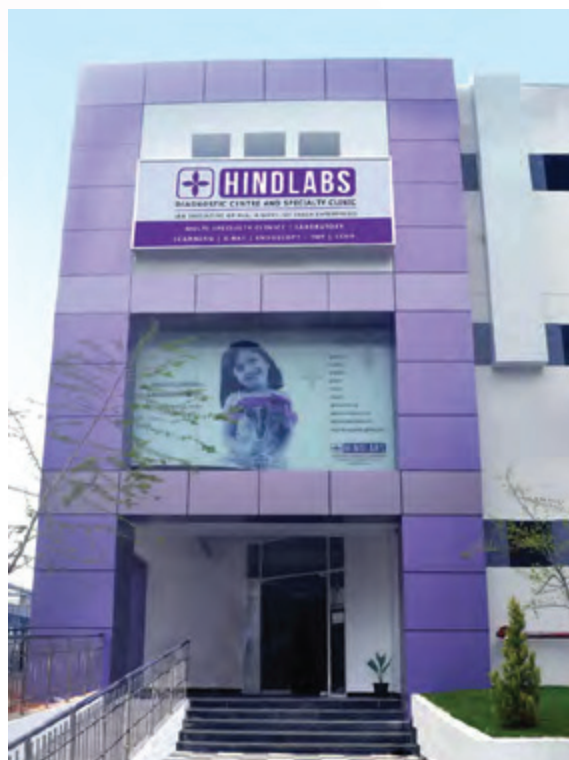
Hindlabs Diagnostic Centre
