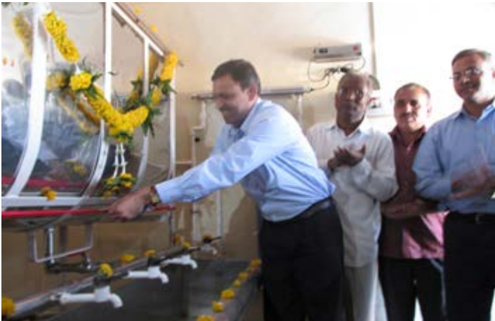
HLL installs a new drinking Water Filtration facility for the Govt. Primary (Kannada - Marathi) School, Kanagala as part of its CSR initiatives on 05 December, 2014.
