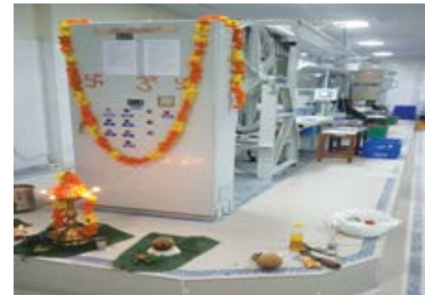
New ETD Machine after Refurbishment installed at KFC on 10 July 2017.
