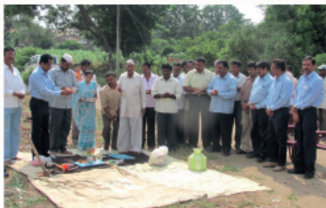
HLL Executives and Kanagala villagers performed pooja at the proposed construction site for toilets at the village
