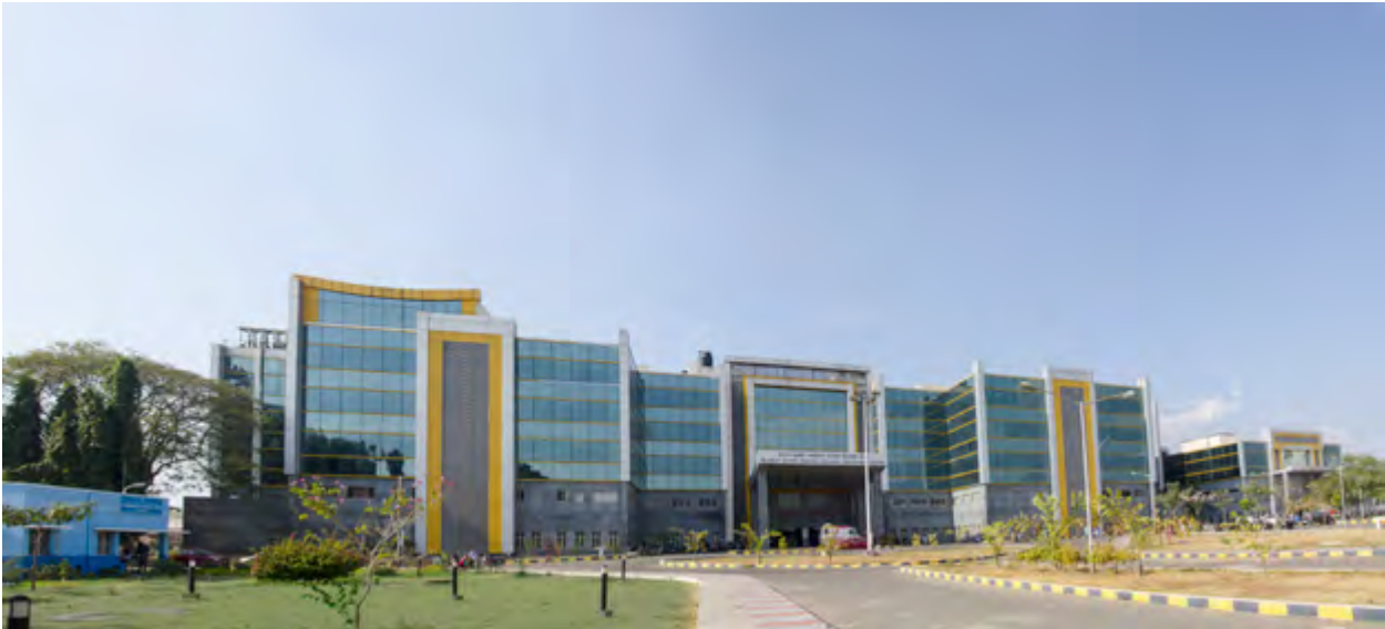
Upgradation of Salem Medical College Hospital, Salem, Tamil Nadu, India.
