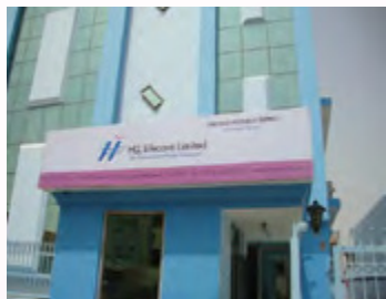
Manesar Facility, Gurgaon
