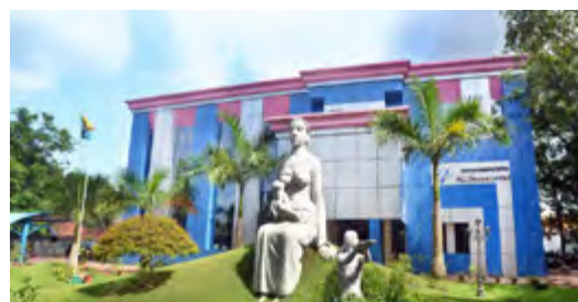
HLL's Corporate headquarters at Thiruvananthapuram, Kerala.
