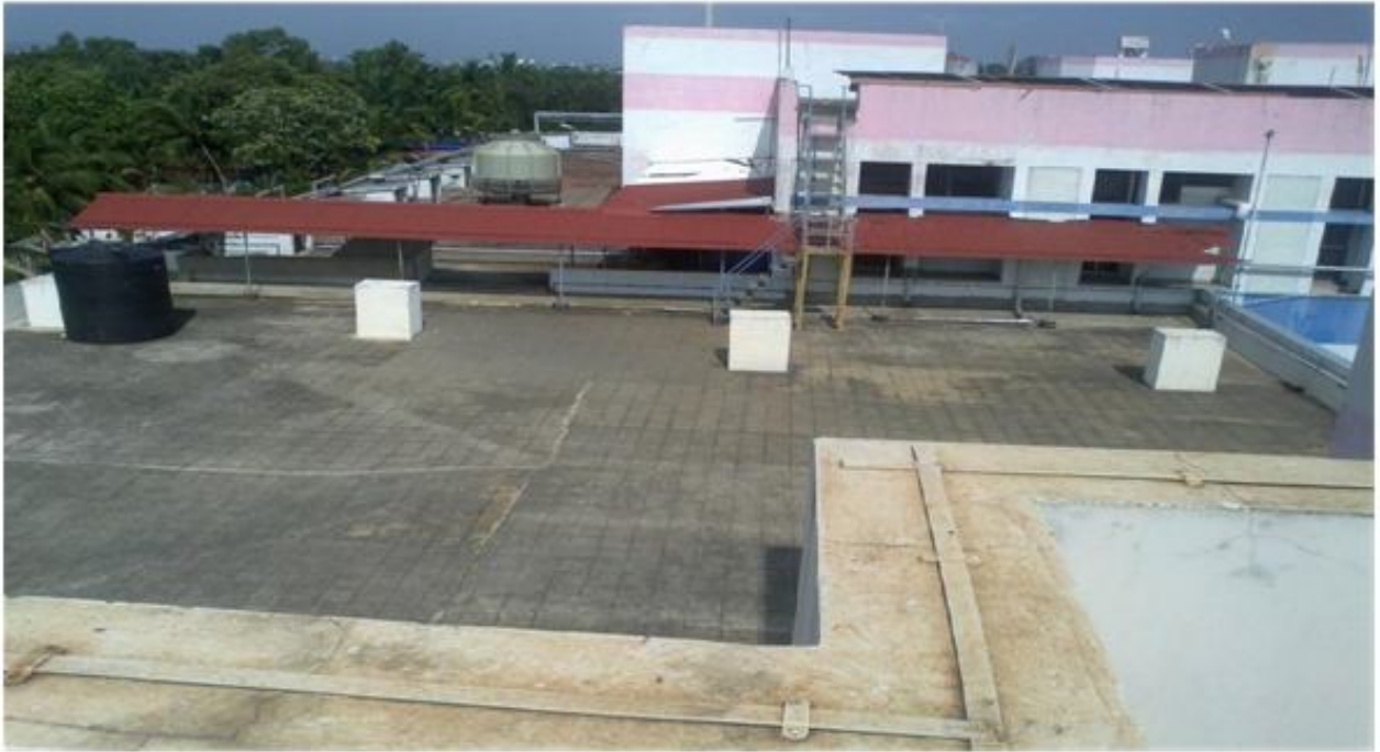
View From top of machine room
