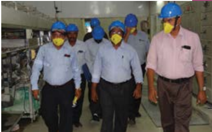
Factories & Boilers Safety Award Judging Committee visits Peroorkada Factory on 26 February 2019.
