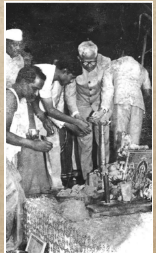
Then Vice President Mr R. Venkataraman laying foundation for the Factory
