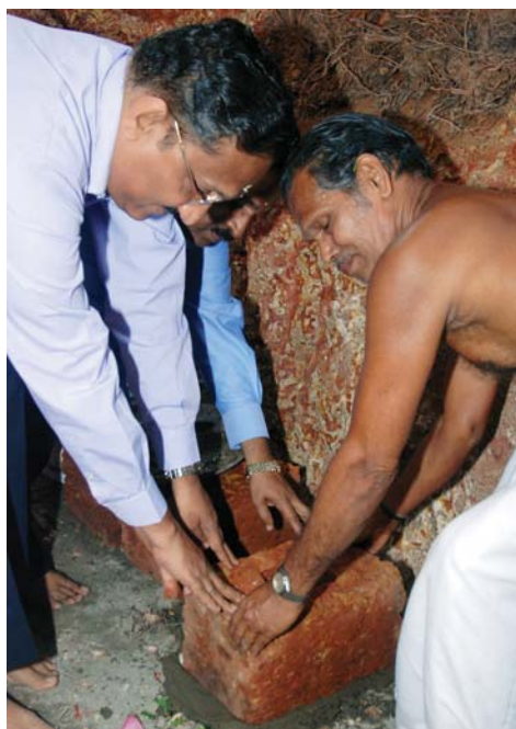
Foundation stone laid for the multi storey building at Kakkanad Factory, Cochin (KFC) as part of the Capacity Expansion Project on 09 May 2011.
